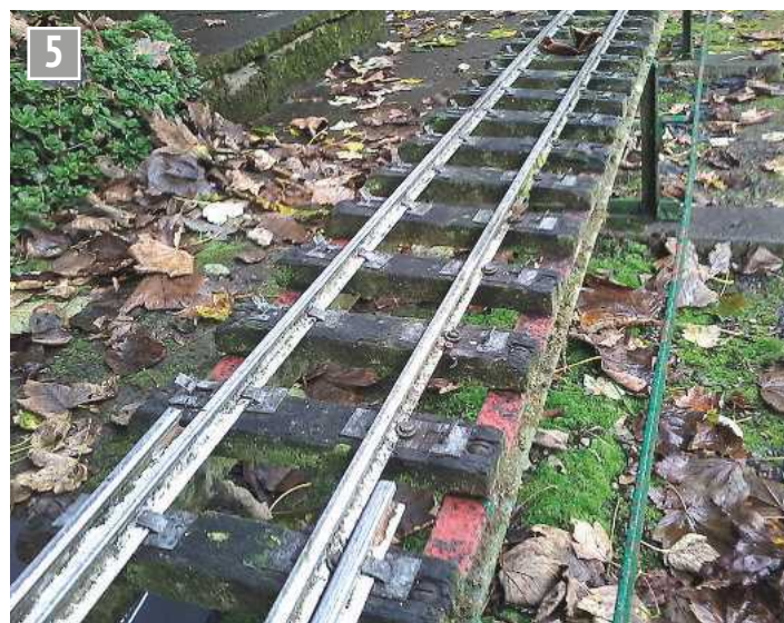
The first rails are removed.
