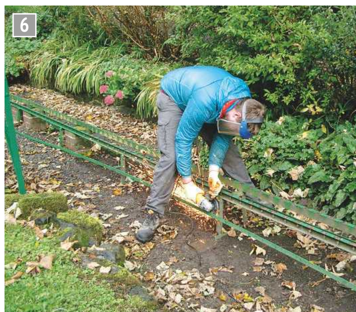
Cutting off the anti-tipping rails for re-use.
