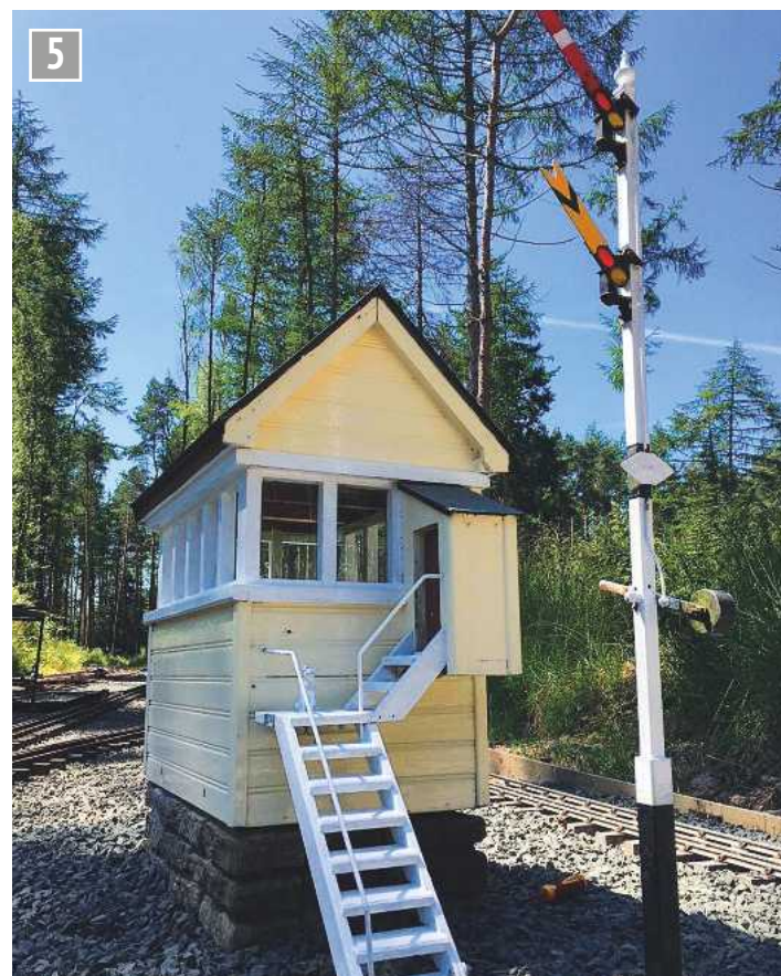
Small signal cabin as above (photo courtesy of Robert McLuckie).
