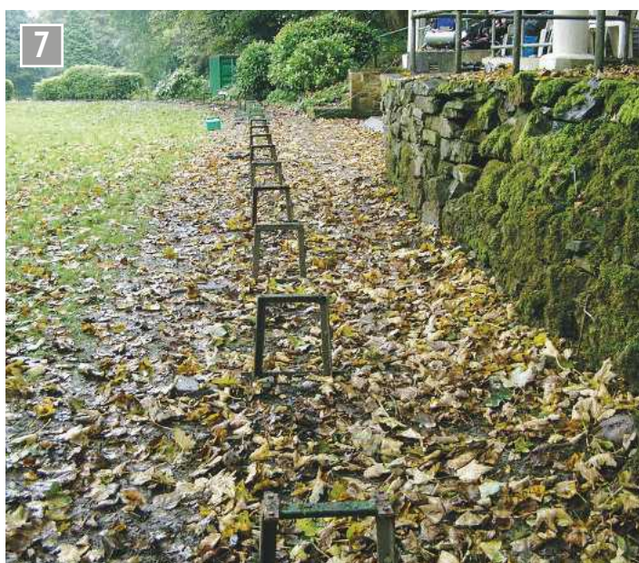
Only the 'A' frames remaining.
