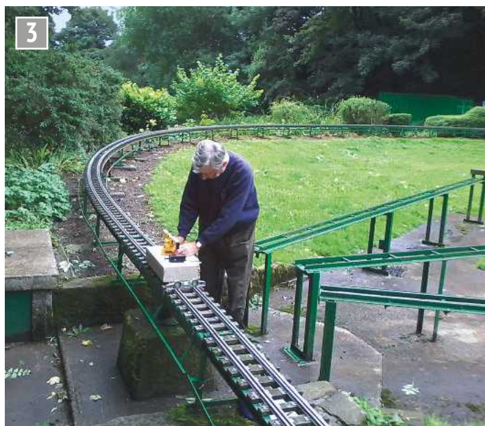
Using the laser alignment tool on the old track.
