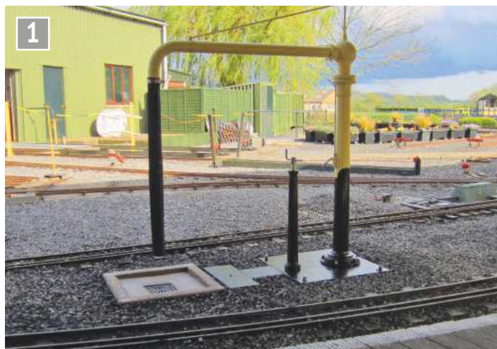
General view of water crane.
