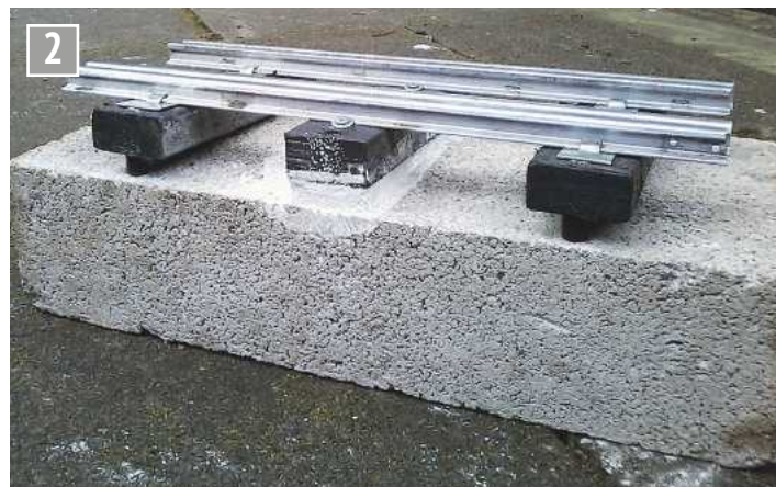
A cement grout is used to prevent the sleeper from moving.
