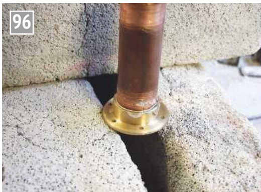
Chimney base ready for silver soldering.
