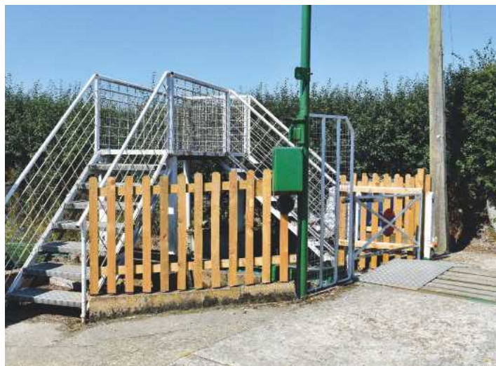
The entrance gate with a good access bridge over the raised track.
