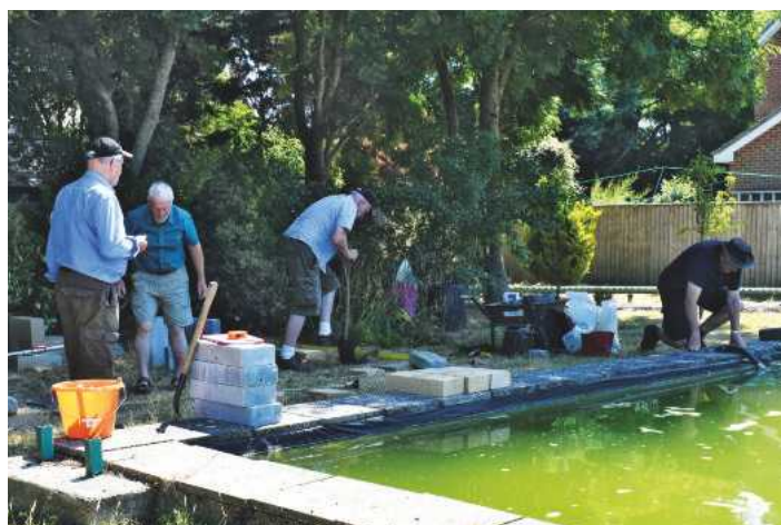
The boat group preparing the base slabs for the new storage shed.
