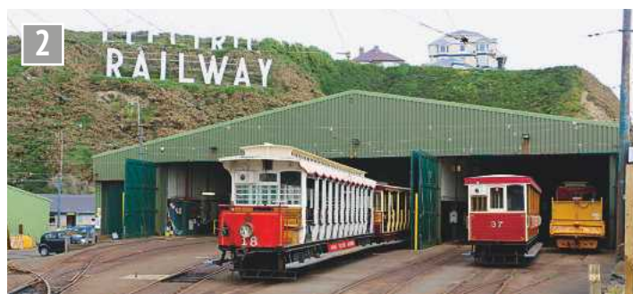
Derby Castle depot and workshops. The Electric Railway sign on the hillside is worthy of Hollywood!
