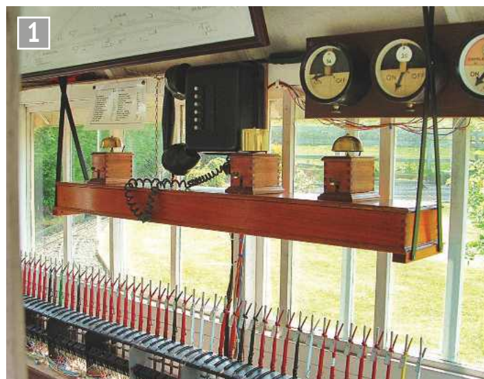
The 48 lever box at Belle Isle.
