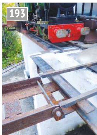
Close up of the top joint and turntable.
