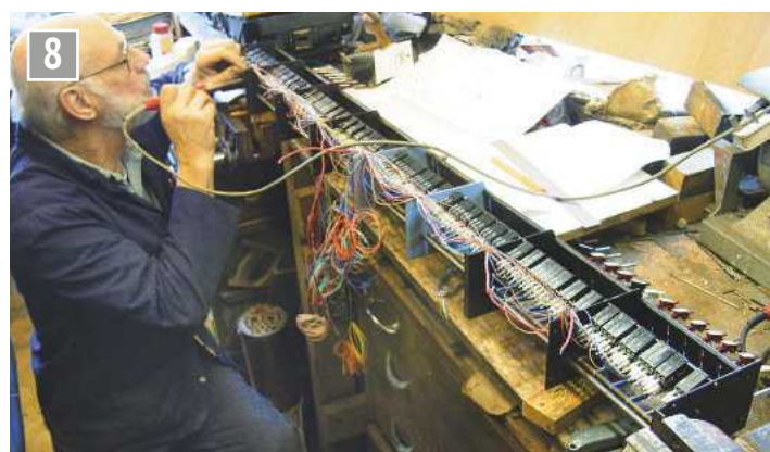
Making the wiring under the frame for Belle Isle Signal Box.
