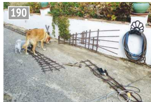
Installation of the three-way point.
