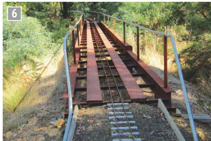
The west end girder bridge.
