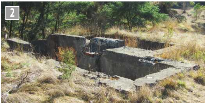
The foundations of the old crushing plant.
