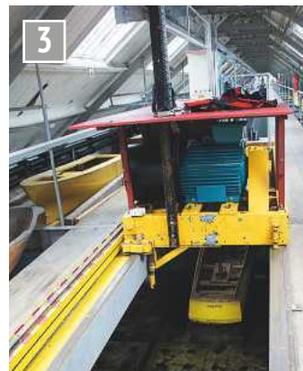
3 View along tank with walkways built over the tank on each side. Tow carriage and electric motor.
