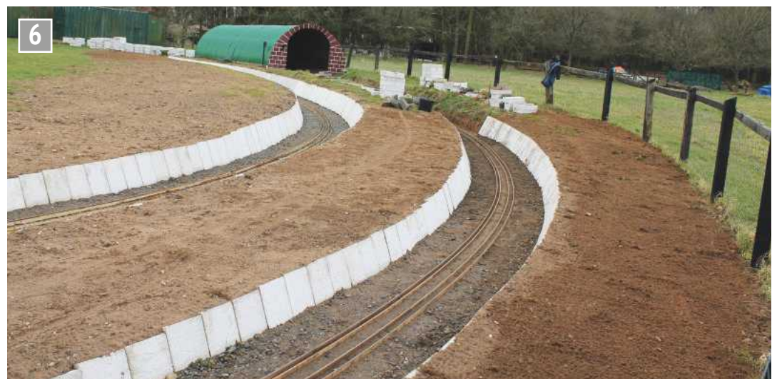
New track at Brandon & DMES (photo courtesy of Mick Wickens).
