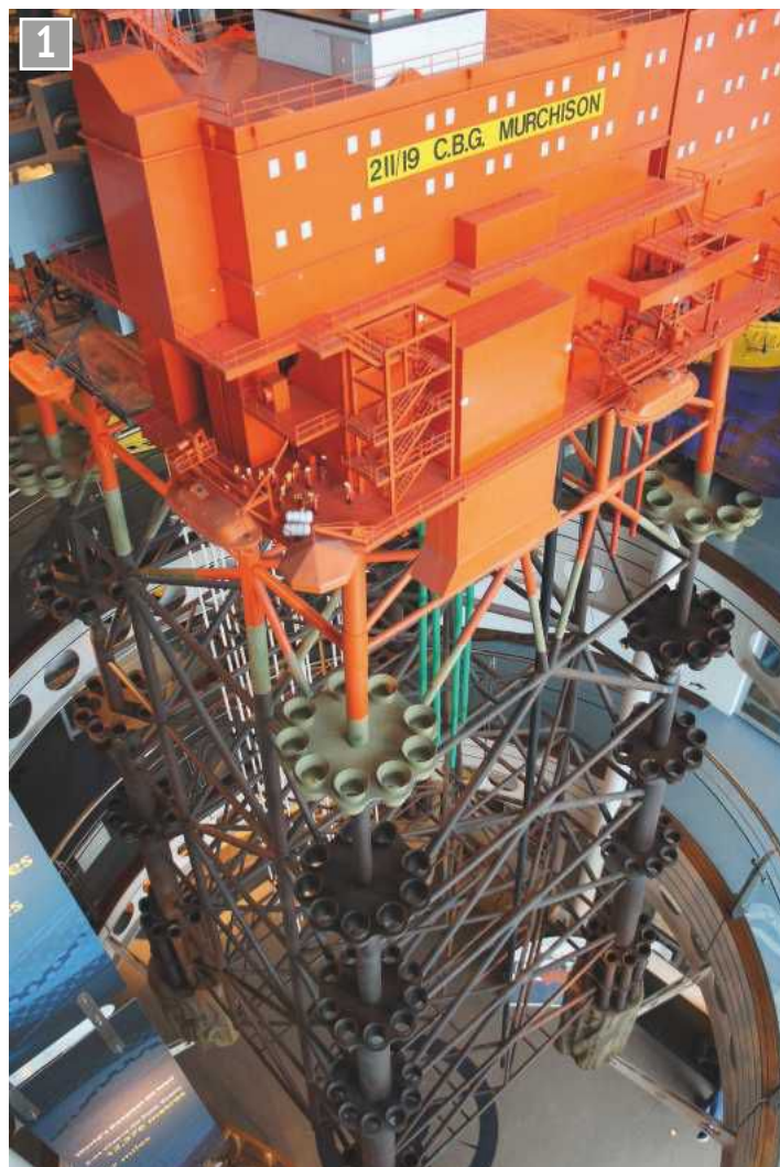
1 Model of the Murchison platform. 254 metres tall, it stands in 156 metres of water. Drilling went down 3275 metres.
