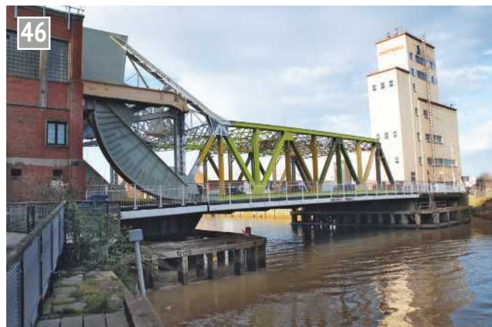
Drypool Scherzer rolling bascule bridge.
