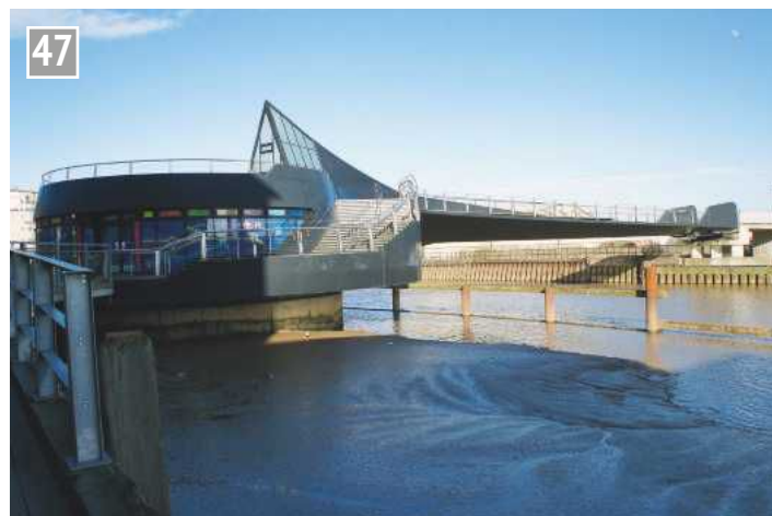
The footbridge rotates like a pinball flipper and carries passengers as it does so.
