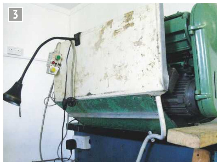
Splashback, lamp and electrical controls.
