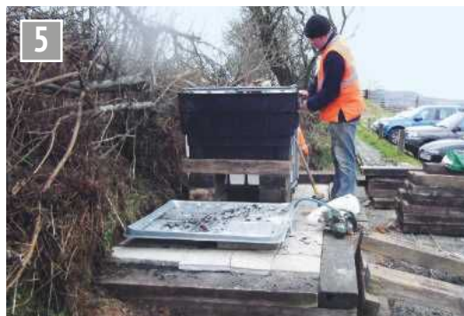
The first tank is installed.
