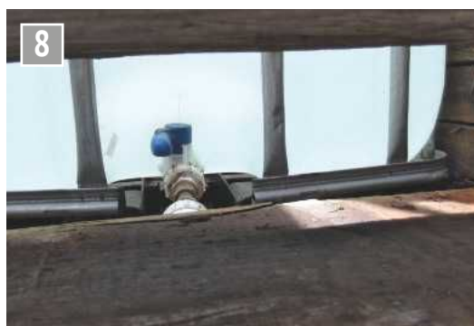
Removing a section of sleeper allows access for isolating a tank.
