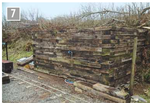
Fully concealed watering facility.
