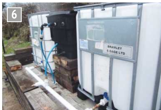
The plumbing is well advanced.
