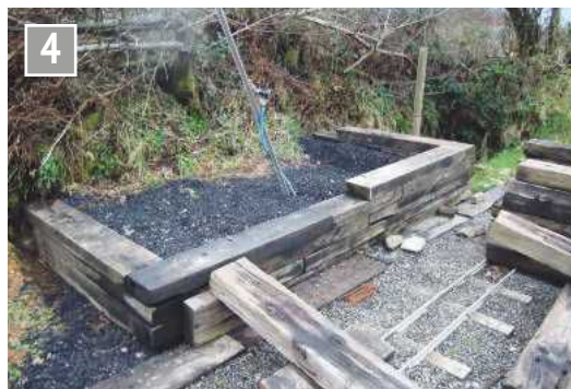
Progress is made with the groundwork.
