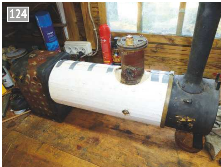
Lagging assembly in place.
