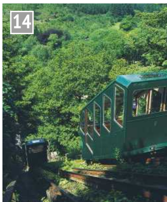
14 Funicular designed by Roger White at the Centre for Alternative Technology, mid Wales. It is ecologically sound using a water balance principle. (Courtesy of Centre for Alternative Technology: www.cat.org.uk )
