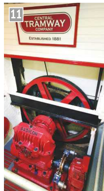
ABOVE: Four winding cables link cars for safety, a fifth cable to the left is a back-up. RIGHT: David Brown Radicon gearbox and motor, disc brake in front and lever operated foot brake just visible behind the sheave or winding wheel. (Courtesy of Central Tramway Ltd.)
