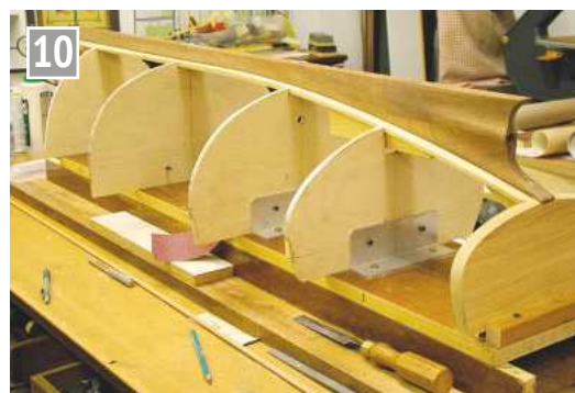
The shadows or moulds were faired using a long spline.
