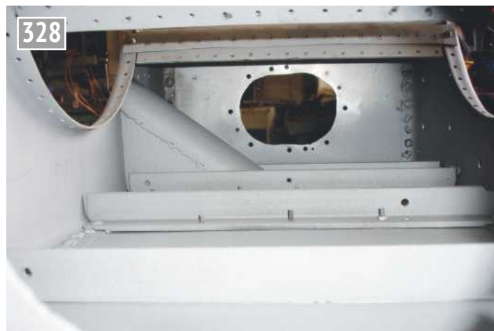
A view inside the completed tank.
