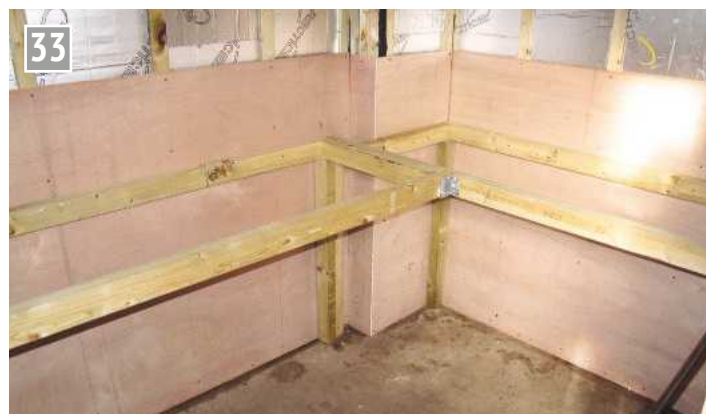
Substantial bench frame work.
