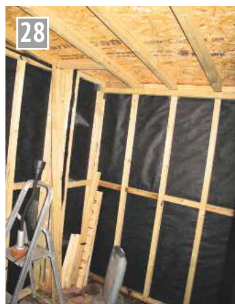
The Sterling board roof.
