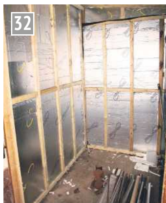
Fully insulated extension.
