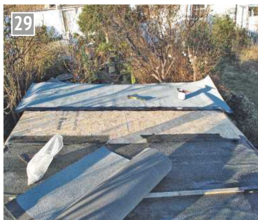
First piece of felt in position.
