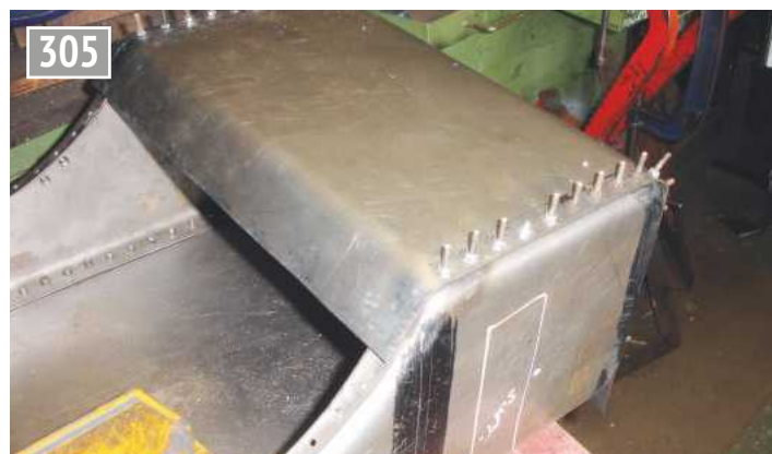
The end/top wrapped and fastened.
