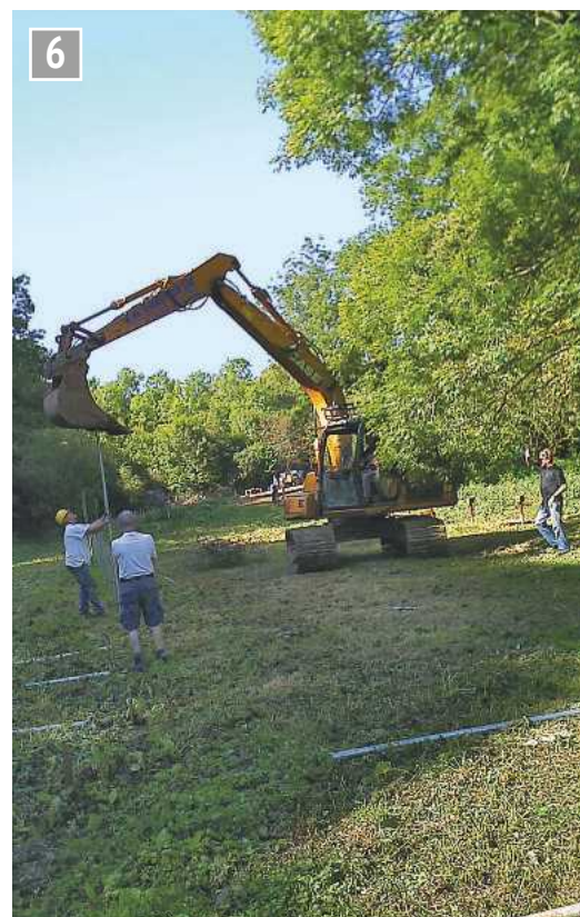
Planting the poles. April 2007.
