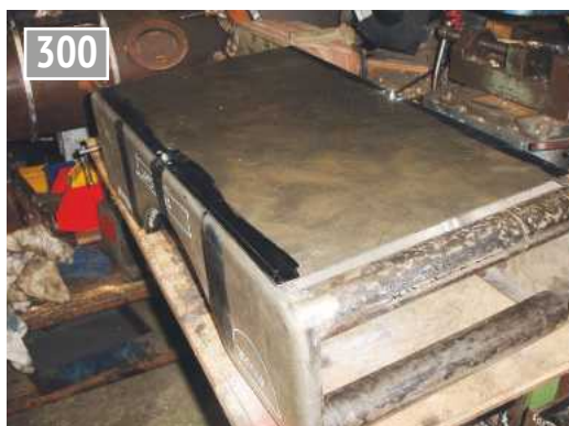
Work in progress on the base plate.
