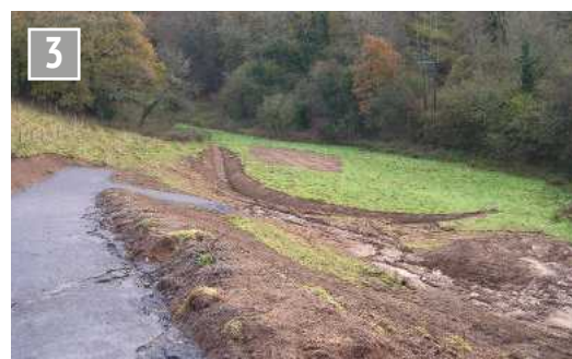
Early access road and the big cutting, December 2005.
