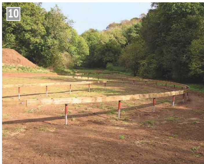
The trackbed planked all round; July 2007.
