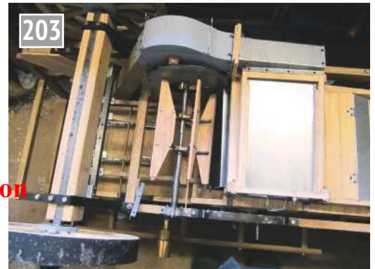
One end plate and the completed fan fitted.
