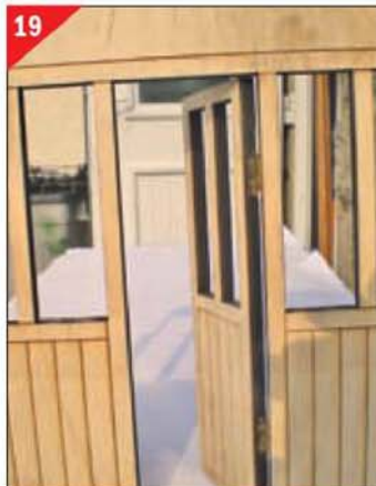
19 The door with hinges fitted, and the glazing bead visible as a brown edge to the windows.
