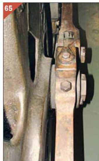
This view is of the large vertical retaining bolt.
