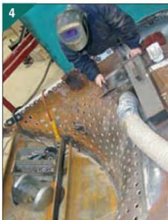
A close-up view of the outer throatplate of the A3 boiler, after replacement of the lower section. (Photo: NRM)
