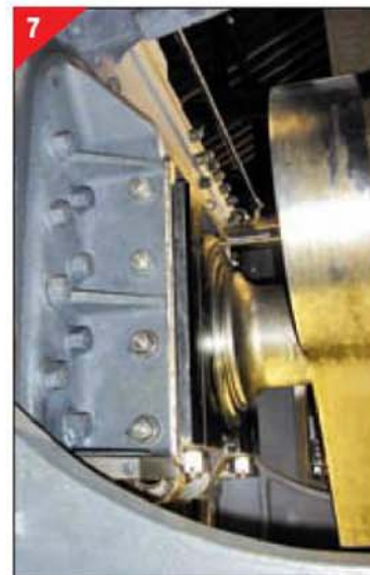
View of a hornblock showing that it is bolted to the frame, not riveted.
