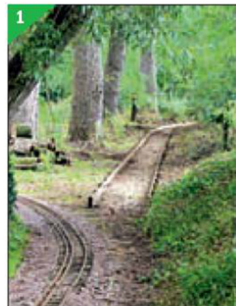
1. The ground level track extension is taking shape at Northampton SME.
