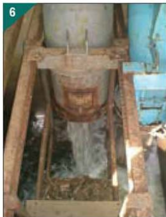
6. Having passed through the turbine the water is exhausted back to the source.
