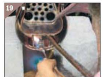
19. Using the oxy-propane lance in the confined space above the firebox.
