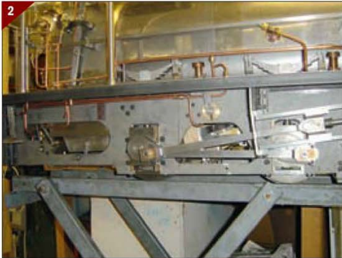
2. Right side pipework from low down, with cab side and sander removed.
