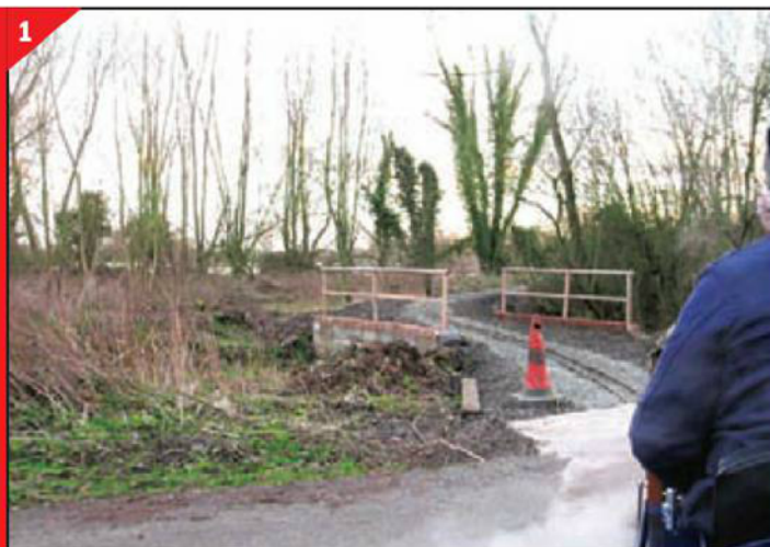
2. Thirstelaine Hall preparing for work.
