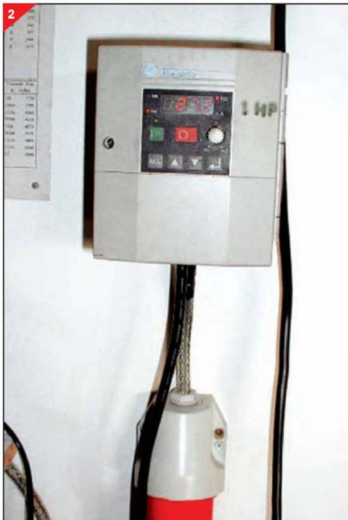
2. One HP Variable Frequency Drive (inverter) used for smaller machines.
