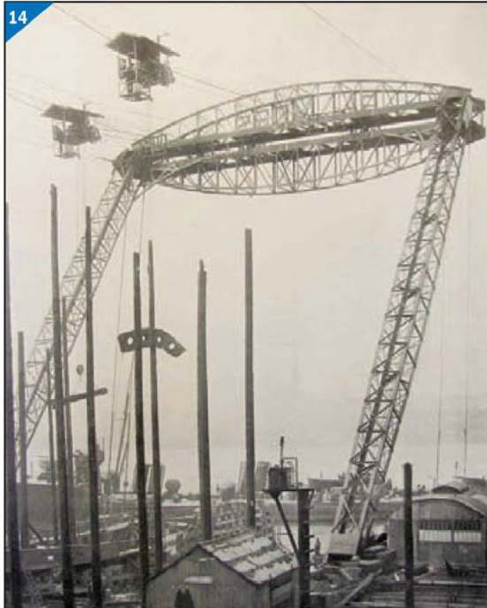
14. Palmers shipyard in Jarrow was home to this complex overhead gantry system serving the slipway area.
