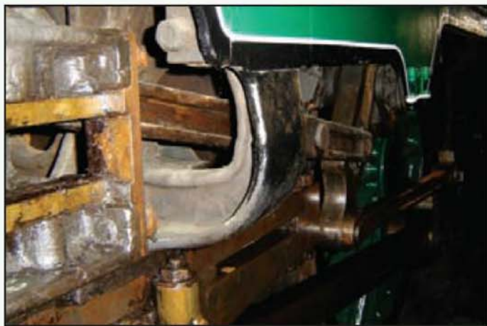
Moving along a little we can see a front view of the slide bar bracket (photo: Derek Tulley).
