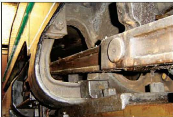
Note the angle iron brackets fitted to hold the rear of the expansion link plate (photo: Derek Tulley).
