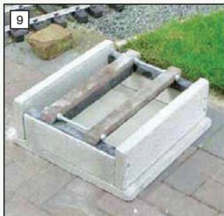
The ash pit before installation. All photos: Tony Finn and Geoff Thorne.
