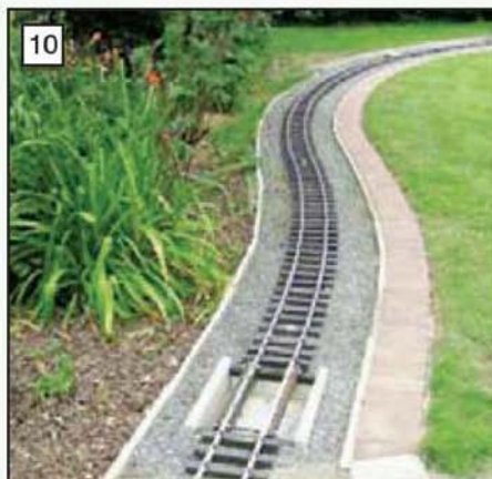
Track laid across the back lawn and the ash pit now installed. The points are not yet built.
