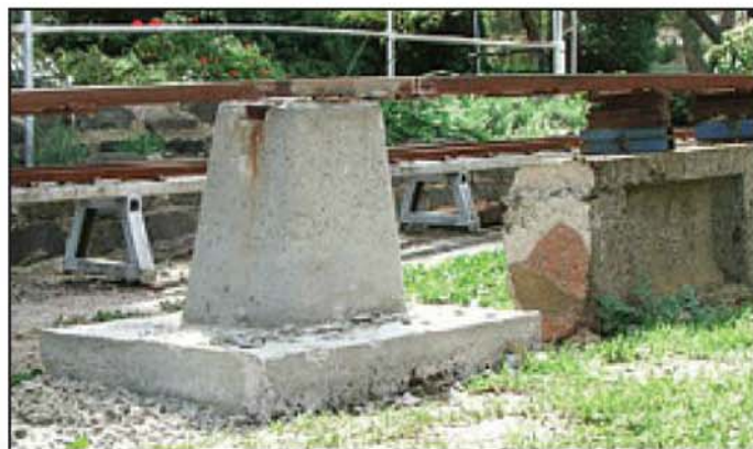
One of the new track pedestals being installed at the Steam Locomotive Society of Victoria track site.
