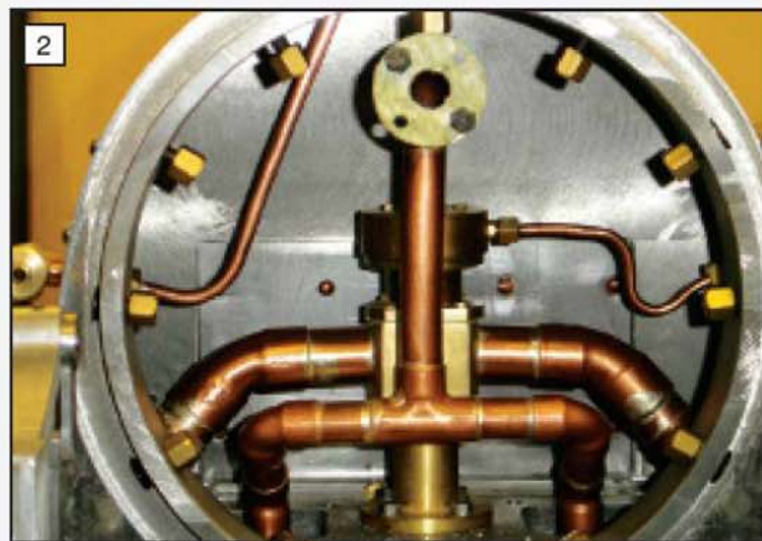
Looking into the back of the smokebox. Note blower and vacuum brake pipework and twelve blind nuts for connecting the boiler.
