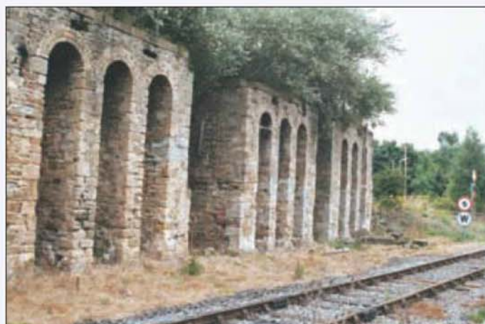
Former coal drops at Shildon - the original traffic for the S&D.
