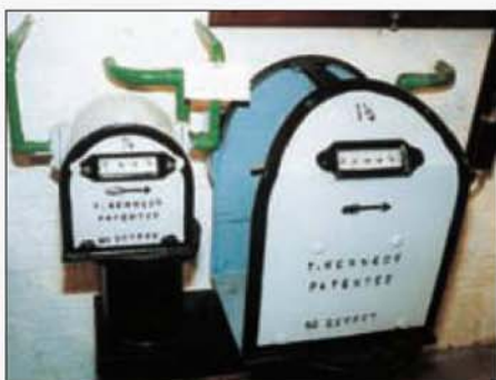
Two Kennedy Water Meters, the right-hand one has its casing removed to show the working parts.
