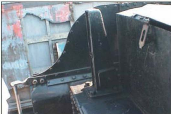
Detail of the coal rail of the 3,500gal. tender at Toddington. Note the angle joining the side and top.
