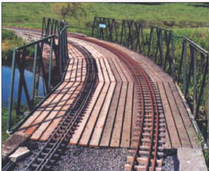
View showing recently widened bridge across stream.
