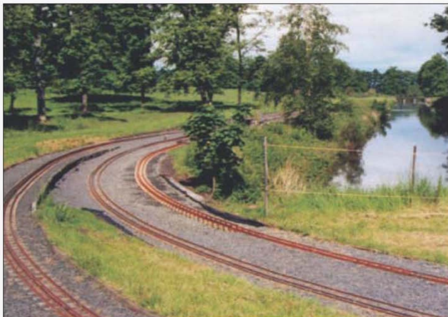
Triple gauge track from steaming bays to the running loops.
