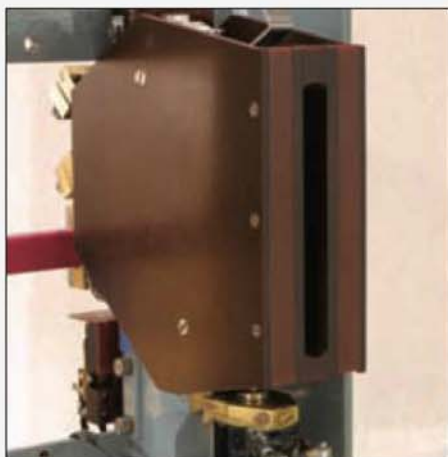
The contactor with arc chute fitted. The arc is discharged through the vertical slot.
