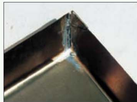
The corner joint from the inside.
