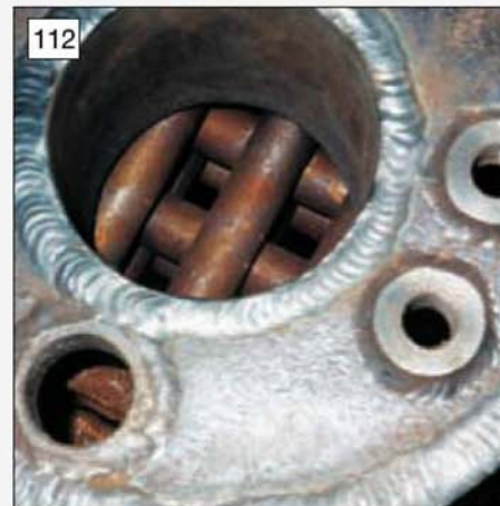
Boiler top plate. Note the inspection hole (photo: John Thompson)
