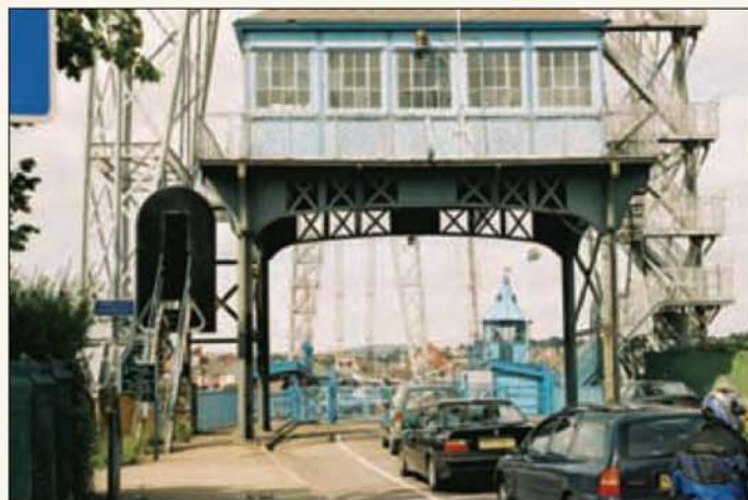
A view of the Motor House on the east side. Cars await their turn to board.
