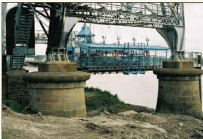
East side foundations - these go 26 metres (81ft.) into the ground.
