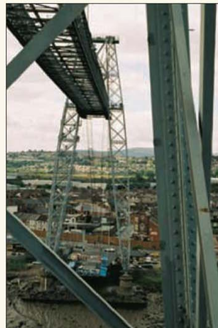
The west tower - it stands 74 metres high.
