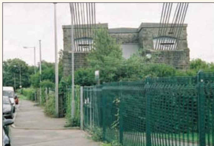
East side cable anchorage holding boom anchor cables.
