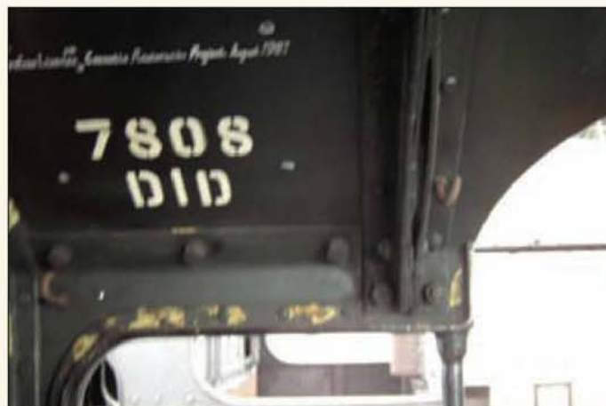
A view inside the cab of Cookham Manor showing the reinforcement used for the sheet metalwork.
