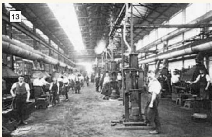
Station Works blacksmith shop with a line of treadle operated steam hammers down the middle of the shop and forges to the left and right.
