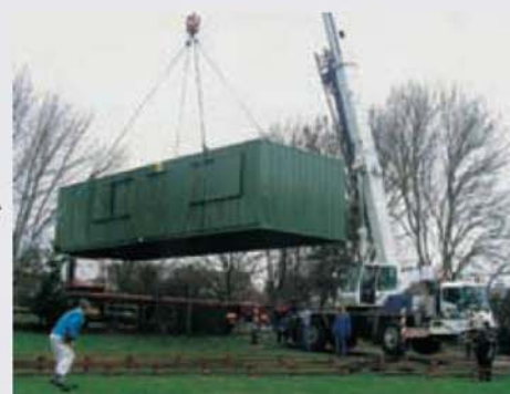
Right: February 2004, the new secure hut arrives on site.
