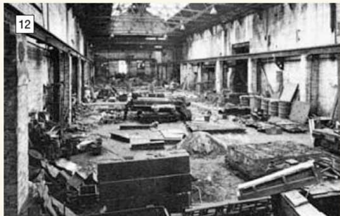
The Garrett foundry looks a demanding place to work. Note the wall mounted rails for the overhead travelling crane needed for heavy lifting.
