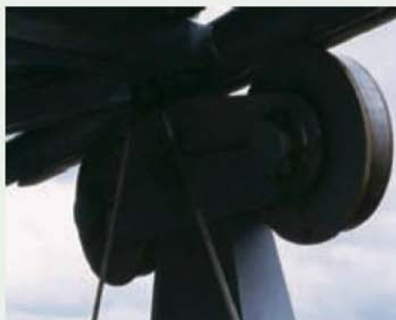
Roller detail of the retractable bridge at Irvine.
