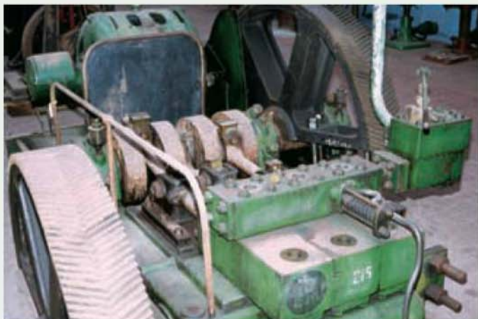
An electric powered hydraulic pump.
