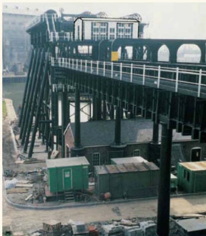
A view from the public grounds looking south-west. The massive upper structure on its five plus five 'A' frames is not functional, although is retained as the structure has 'Ancient Monument' status. For safety, the massive balance weights and wire ropes have been removed but are on display.
