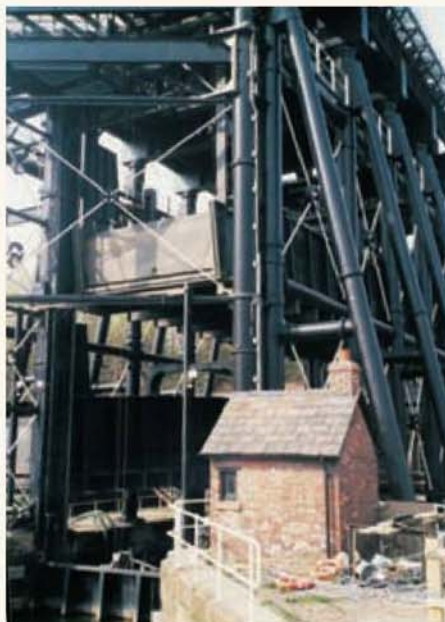
The right-hand caisson is on its way down. The brick hut was originally for the toll collector. The sloping 'A' frames support the 1908-1983 winding system which serve no function today.
