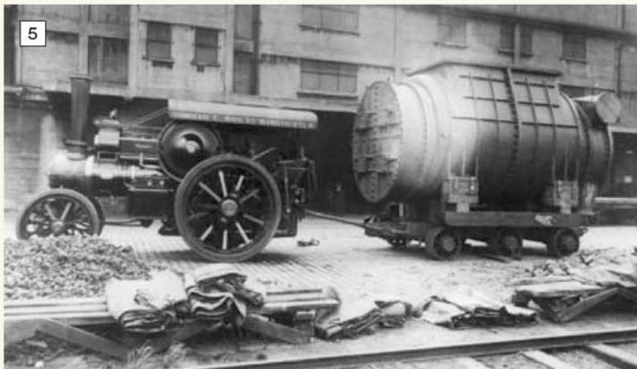
5 Talisman with a 60 ton condenser en route to Manchester docks. Note scotches under trailer wheel and large pulley block lying in the road between engine and load.
