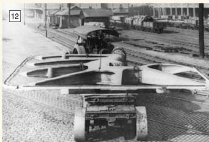
Titan with a 24ft. wide rudder casting for HMS Rodney from Cammell Laird & Co. Ltd., Sheffield, here pictured at Manchester docks in 1924.
