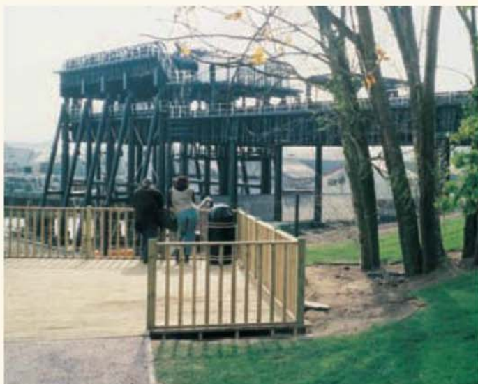
A view south from the upper basin, along the aqueduct. The 1875 brick boiler and pump house is under the aqueduct. Note the control cabin over the end of the aqueduct. Landscaping of the site is now almost complete.
