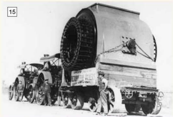
Vulcan and Titan haul a 90 stator destined for Manchester Corporation electricity works. Note that even on apparently level ground the trailer wheels have been scotched.
