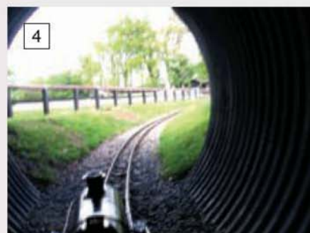
The tunnel is 6ft. wide and on a right hand curve.
