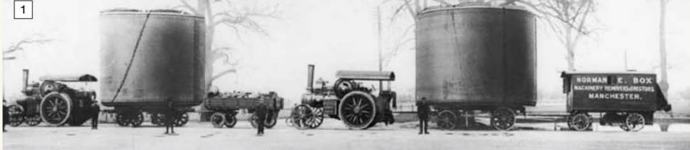
An atmospheric shot of NEB's Fowler B6 road locomotives Titan and Vulcan, each with a 45 ton marine boiler en route from Newcastle to Southampton in 1919. Titan has a coal wagon in tow and Vulcan the crews' living van.
