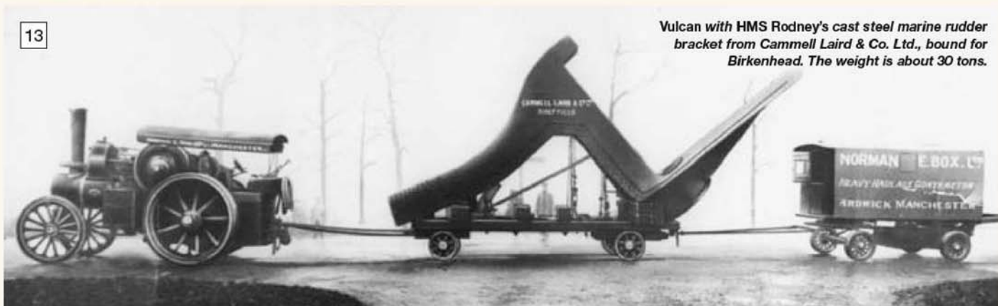
The NEB photos contain a number of shots taken in 1924 of parts in transit for HMS Rodney. Here one of the two cast steel propeller shaft brackets is being moved. Each bracket weighs 35 tons.
