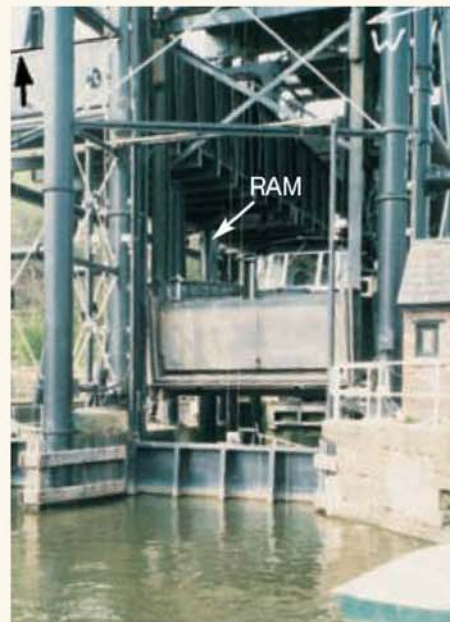
The trip boat is descending the 50ft. 4in. from the Trent & Mersey Canal to the River Weaver. Note the 3ft. dia. ram under the left hand caisson. Its ceramic coating protects it against corrosion.
