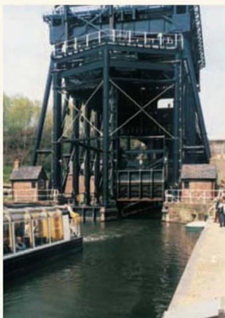
The Anderton Lift viewed from the south. The right-hand caisson gate is closing after the trip boat has left on its way into the River Weaver.
