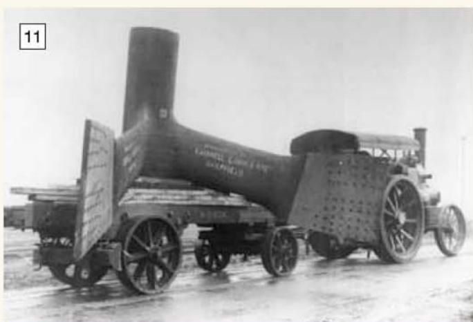
The NEB photos contain a number of shots taken in 1924 of parts in transit for HMS Rodney. Here one of the two cast steel propeller shaft brackets is being moved. Each bracket weighs 35 tons.
