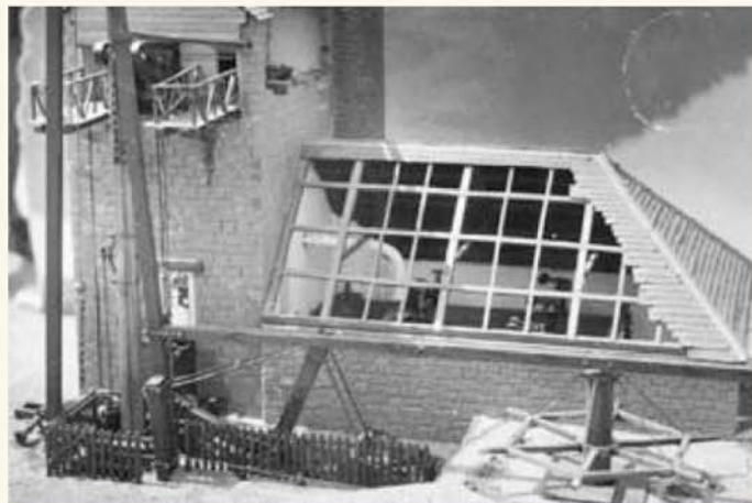
A closer view of the pump shaft and operating beam. The tiles on the roof of the boiler house have been omitted to give visual access within.
