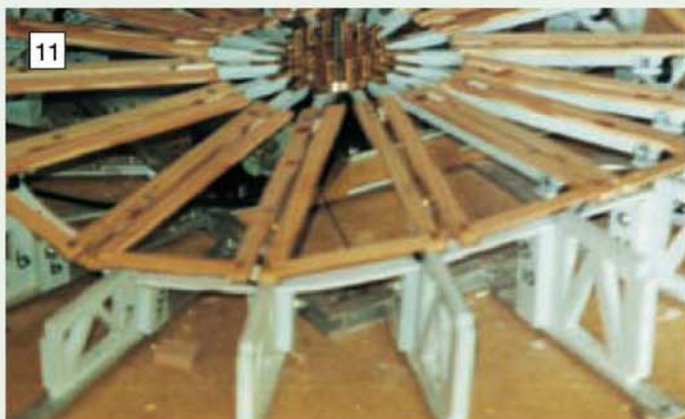
Slave bars maintain uniform spacing between the wheel bars.
