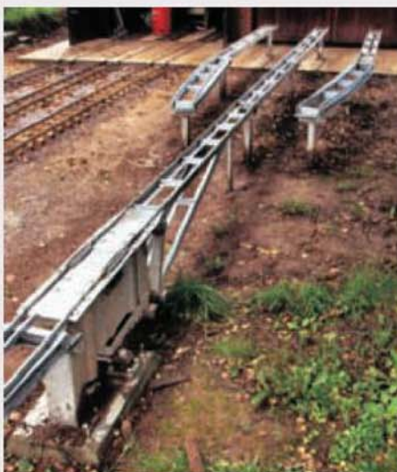
The configuration of the swing beam track is evident from this general view.
