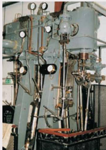
A Fleming & Ferguson of Paisley inverted two-cylinder cross-compound vertical engine of 1942 is from an Admiralty crane ship.
