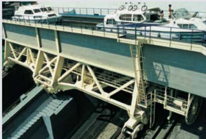
The trough with its supporting structure and bogies. These boats spent some time stuck here while a minor technical problem was sorted out.
