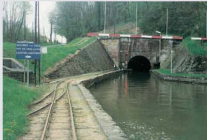
The tunnel mouth with a short section of the old narrow gauge haulage railway used to pull the barges.
