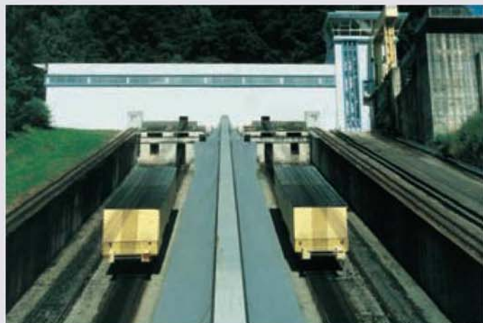
Looking up the lift towards the machinery room and upper gate structure. The two counterweights are descending. There is room for two more either side.
