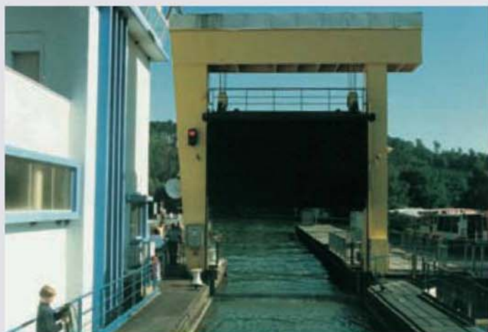
The upper gate open ready for departure. The boat on the right is moored in the entrance for the possible future second gate.
