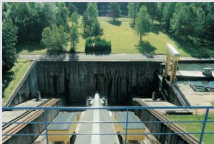
Looking down the lift showing the lower gate. The provision for an extra gate can be seen.
