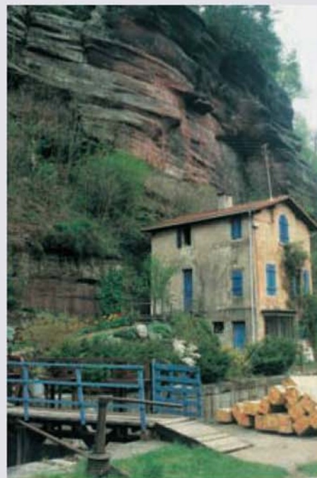
A lock keeper's cottage beside one of the seventeen locks replaced by the lift. The timber gives some hope that it may be intended to rewater this section of the canal, which would look better even if not navigable.
