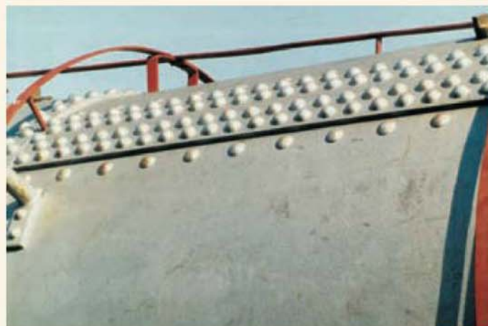
Boiler barrel detail. Note the cover plates inside and out and the crinolines for the lagging and outer casing.
