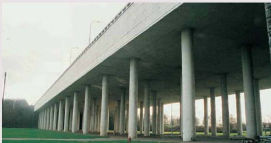
The substantial aqueduct leading from the summit section of the canal to the Ronquieres gate structure is supported on a forest of columns.
