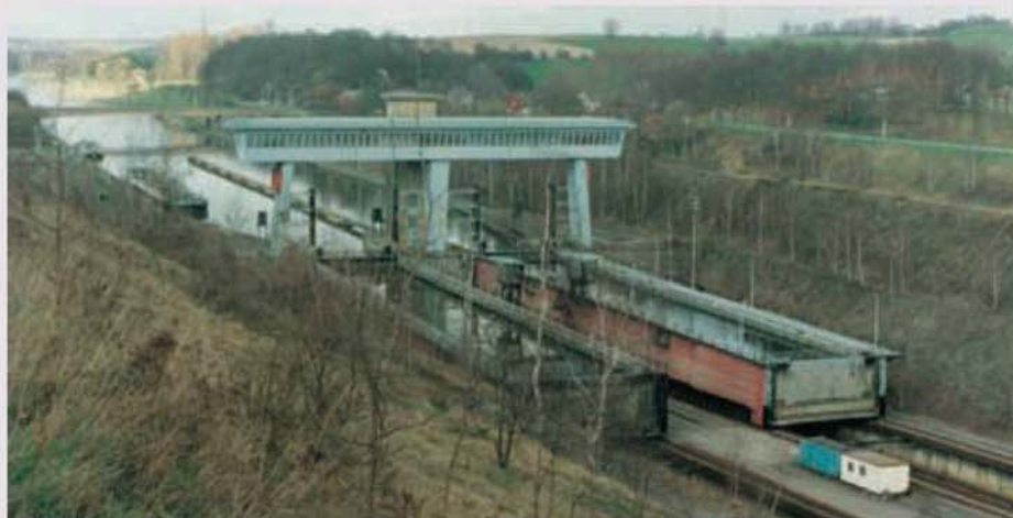
In this winter view of Ronquieres the troughs can be seen in the lower position.
