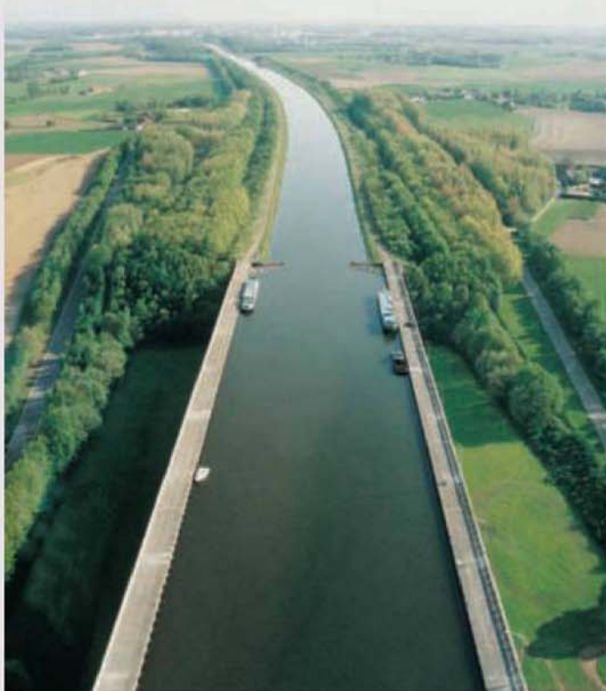
Looking down the inclined plane from the tower. This is railway engineering on a grand scale. There are two sets of rails on each side, one for the troughs and the other for the equally heavy counterweights.
