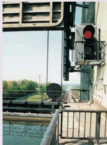
The gate at the top of the incline. The extra gate in the raised position is used to permit work on the working gates when required.
