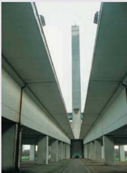
An interesting perspective showing the Ronquieres viewing tower framed between the raised part of the inclined planes.
