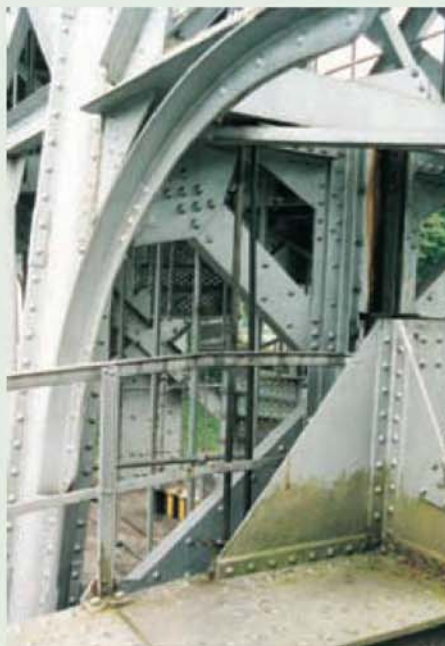
Detail of the ironwork - there are plenty of rivets to count here!
