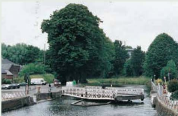
A manually operated opening bridge between the shiplifts in La Louviere.
