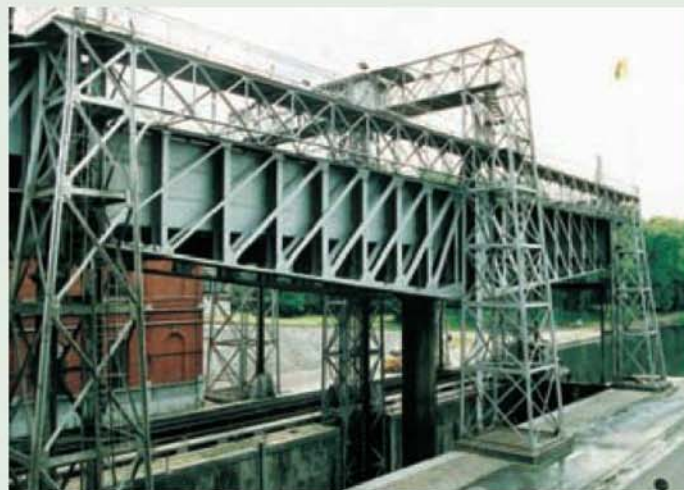
The top lift near Cantine des Italiens, showing the hydraulic ram.
