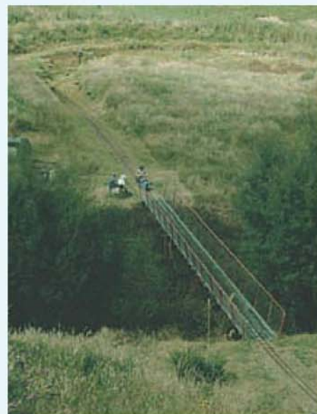
A view from the boundary fence looking down on one of two major bridges.
