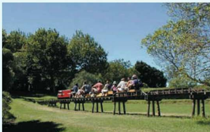
The viaduct at Manakau Live Steamers near Auckland.
