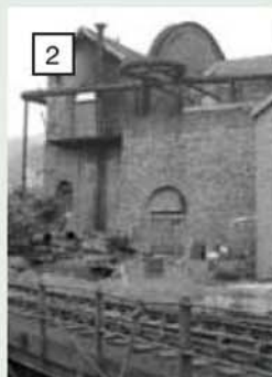
The 44ft. diameter Waddle fan used to ventilate the coal workings in Deep Duffryn, Mountain Ash.
