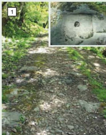
Stone blocks on which the cast iron rails rested on the Merthyr Tramroad. The inset shows one of the stone blocks with spike hole.
