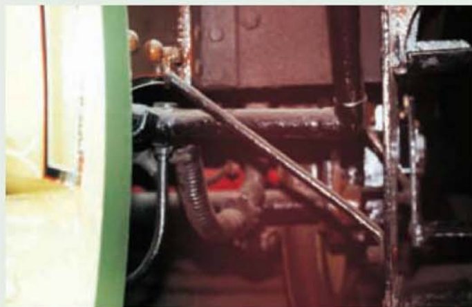
H.R. No. 103 cab steps viewed from the front showing the bracing strut.
