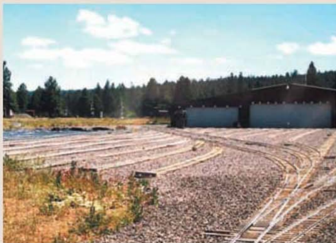
Ladder Sidings beside workshop.
