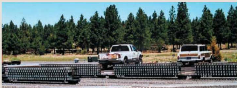
Piles of track on tracklaying train.
