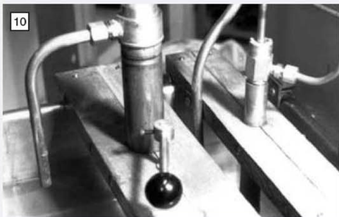
The black knob on the pit pump closes off the inlet valve to put a load on the pump and slow the engine down. The smaller pump feeds the cistern.
