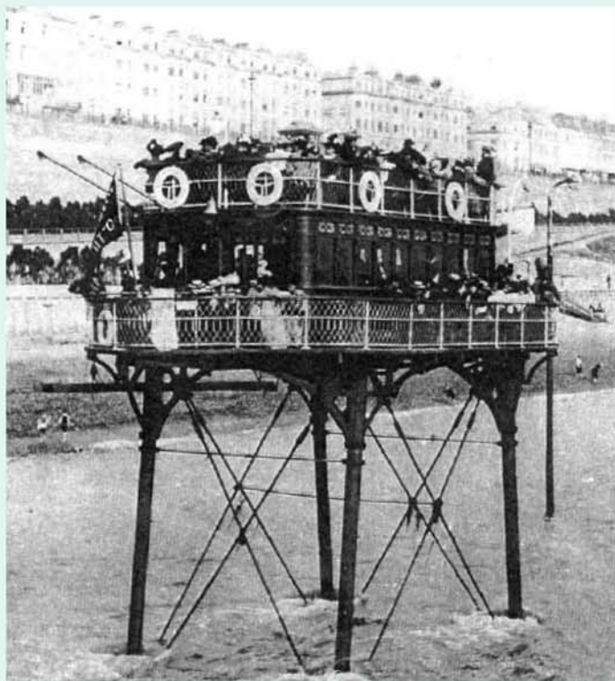
Pioneer with the tide 'on the turn', the sponsons only just about covered and seaweed hanging from the cross braces.
